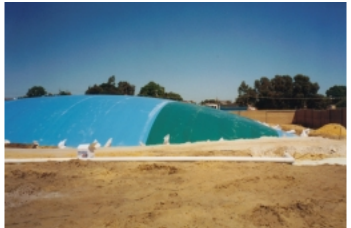
PAH contaminated soil bioremediation using the FABCOM® biosystem
